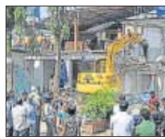
BMC conducts a demolition drive on Wednesday.
